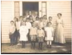
Banks North Class Photo (FF_Schools_Elementary_Banks North_03)
