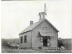
Wilson's Mill school building (FF_Schools_Elementary_Wilson_01)
