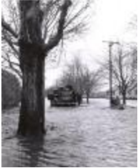
Hurricane of 1953 - Beach Road (FF_Hurricane1953_F1_001)
