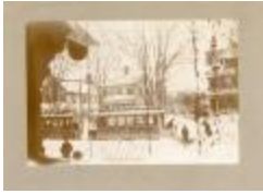
Park Avenue Trolley (BP_Transittrolleys_001)
