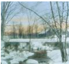
Aspetuck Mill Dam (MOW_125_Aspetuck Mill Dam-Winter)
