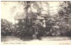
Benson Tavern, Fairfield, Conn. (PC_FF_Houses_Benson_01)
