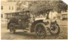
Fire engine (FF_FireDept_Co-1_F2_01)
