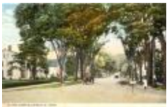
Flints Corner, Fairfield, Conn. (PC_FF_Streets_Flints_01)
