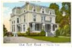
Unquowa Hotel, Fairfield, Conn. (PC_FF_Hotels_Unquowa_01)
