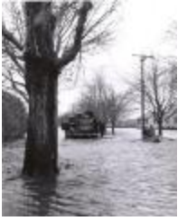
Hurricane of 1953 - Beach Road (FF_Hurricane1953_F1_001)
