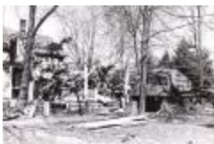
Hurricane of 1954-Clearing Rubble (FF_Hurricane1954_001)
