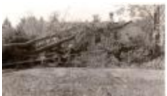
1938 Hurricane Fairfield trees and wires down (FF_Hurricane1938_F1_030)
