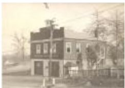
Tunxis Hill Fire Dept. (FF_FireDept_Co-2_01)
