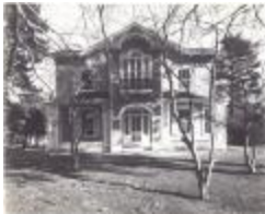
415 Old Post Road (FF_BLDGS_415Old Post Rd_3)
