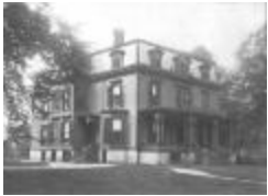
808 Old Post Road (FF_BLDGS_808Old Post Rd_2)
