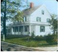
Redfield House (MOW_105a_Redfield House-Mill Plain)
