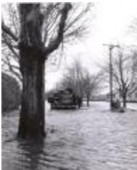
Hurricane of 1953 - Beach Road (FF_Hurricane1953_F1_001)
