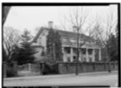
739 Old Post Road (FF_BLDGS_739Old Post Rd_1)
