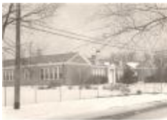
Grasmere School Building (FF_Schools_Elementary_Grasmere_02)
