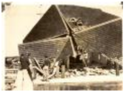
Hurricane of 1938 - Destroyed Home (FF_Hurricane1938_F1_001)
