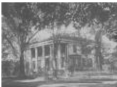
458 Old Post Road (FF_BLDGS_458Old Post Rd_4)
