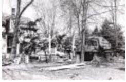
Hurricane of 1954-Clearing Rubble (FF_Hurricane1954_001)
