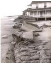
Hurricane of 1954-Fairfield Beach Damage (FF_Hurricane1954_004.tif)
