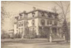
808 Old Post Road (FF_BLDGS_808Old Post Rd_06)
