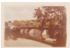
Preston Bridge, Norwich, CT. (Photographs Fold. 009 Photo 167)
