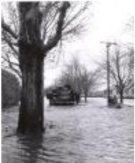
Hurricane of 1953 - Beach Road (FF_Hurricane1953_F1_001)
