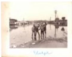
1979 Flood, near 3379 Post Road (FFCN_Floods_1978_1974_1980_1989 (8))
