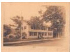
Photographs - Exterior View of Allis-Bushnell House in 1924 from the Allis-Bushnell House Exterior and Interior Views Photo Album (A2023.ABHouseViews.001ab)
