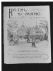
556 Old Post Road (FF_BLDGS_556Old Post Rd_5)
