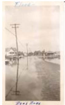
1938 Hurricane Reef Road flooded (FF_Hurricane1938_F1_028)
