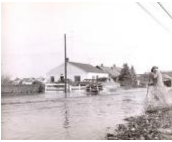
Hurricane of 1953 - Reef Road (FF_Hurricane1953_F1_004)
