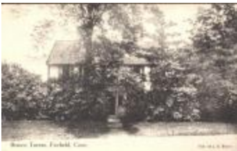
Benson Tavern, Fairfield, Conn. (PC_FF_Houses_Benson_01)
