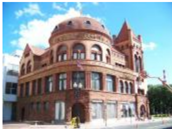
Structure: Barnum Institute of Science and History (1893.000.001)
