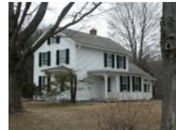
CD - Revisiting the Historical and Architectural Survey of Madison CD#1, Cope Road (A2004.HistSurv.001.CopeRd)
