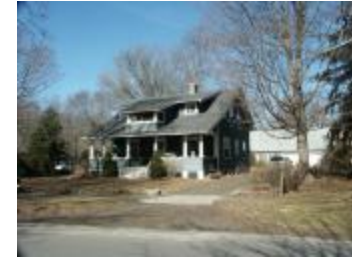
CD - Revisiting the Historical and Architectural Survey of Madison CD#1, Britton Lane (A2004.HistSurv.001.BrittonLn)
