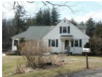
CD - Revisiting the Historical and Architectural Survey of Madison CD#1, County Road (A2004.HistSurv.001.CountyRd)
