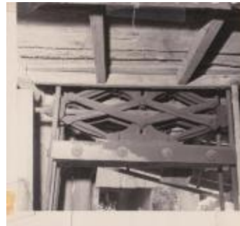
interior view, Lewis Mill (Photographs Fold. 007 Photo 144-2)
