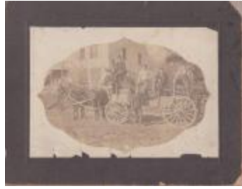
Line crew building first telephone line in Preston (Photographs Fold. 003 Photo 063)
