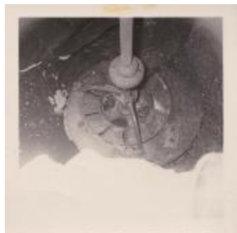
interior view, Lewis Mill (Photographs Fold. 007 Photo 140)
