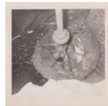
interior view, Lewis Mill (Photographs Fold. 007 Photo 139)
