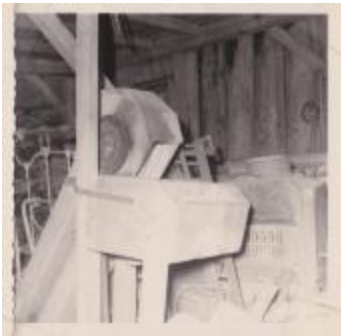
interior view, Lewis Mill (Photographs Fold. 007 Photo 144-3)
