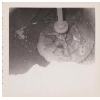
interior view, Lewis Mill (Photographs Fold. 007 Photo 138)
