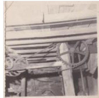
interior view, Lewis Mill (Photographs Fold. 007 Photo 144-5)
