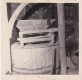
interior view, Lewis Mill (Photographs Fold. 007 Photo 143-1)
