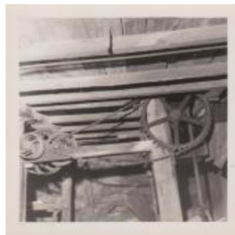
interior view, Lewis Mill (Photographs Fold. 007 Photo 142)
