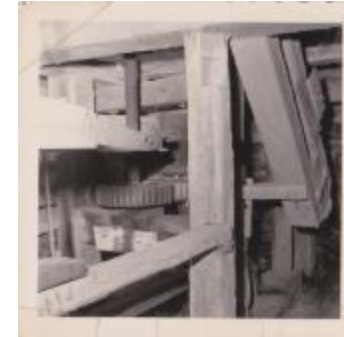
interior view, Lewis Mill (Photographs Fold. 007 Photo 144-1)
