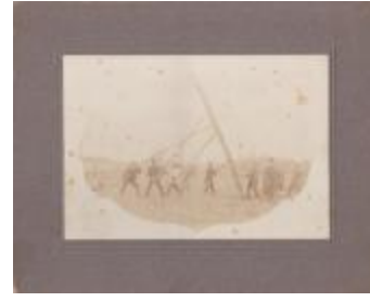
telephone company crew installing lines (Photographs Fold. 007 Photo 151)
