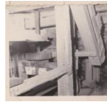
interior view, Lewis Mill (Photographs Fold. 007 Photo 144-6)
