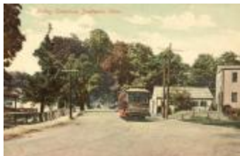
Trolley Terminus, Southport, Conn. (PC_SP_Streets_Trolley_01)
