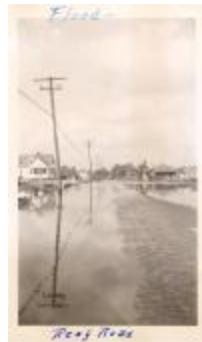
1938 Hurricane Reef Road flooded (FF_Hurricane1938_F1_028)
