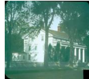
Burr Homestead (MOW_133a_Burr Homestead-wall)
