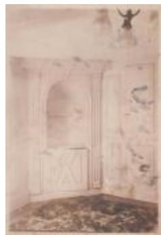
interior view, Captain John Williams home (Photographs Fold. 002 Photo 053)
