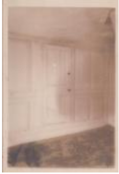
interior view, Captain John Williams home (Photographs Fold. 002 Photo 056)
