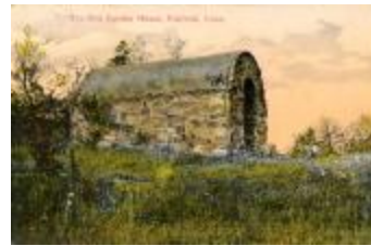
The Old Powder House, Fairfield, Conn. (PC_FF_Powder House_01)
